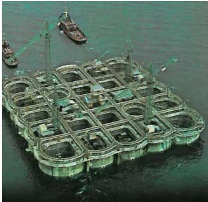
FIGURA 4.4 - Transporte dos Tanques.
